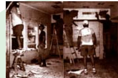
The volunteer renovations crew working at 1601 W. Alabama.
